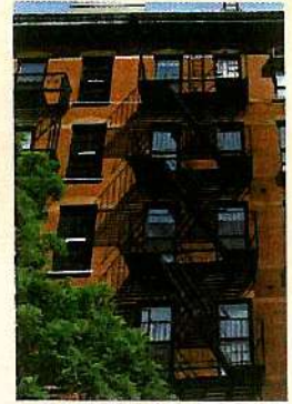
6 a fire escape
